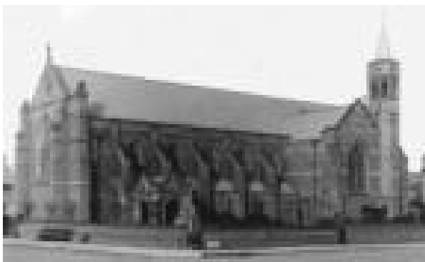
St Faith's in 1937 showing how the roads had developed around the church.
