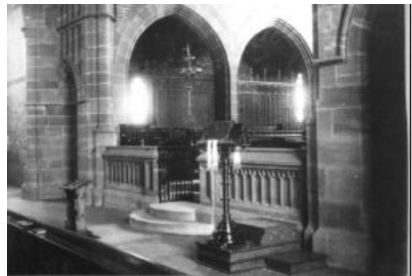
The Chancel before the screen was fitted in 1921. The gas lighting is evident.
